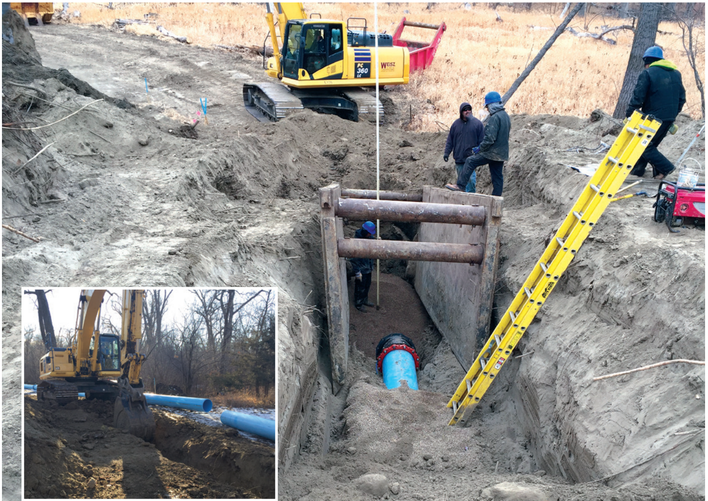
Trenching and pipe installation.
